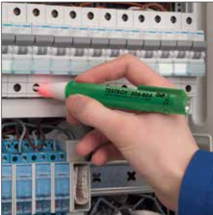
Testboy illuminates with voltage present
